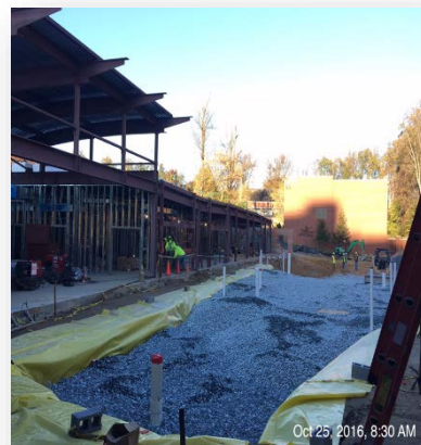
Stormwater management structure under playground
