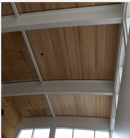
Cedar in multi-purpose room ceiling
