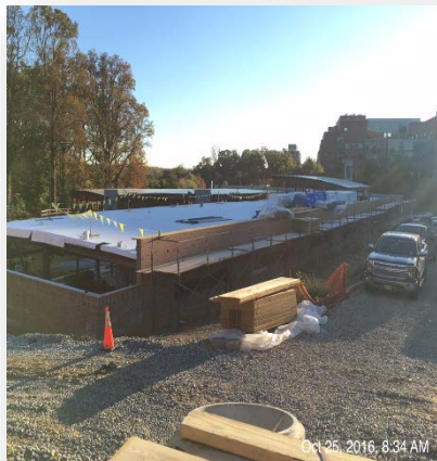
Brick work and masonry install (October 2016)
