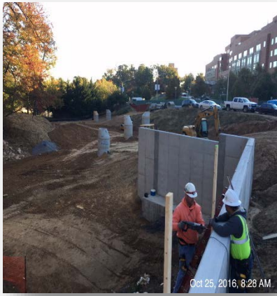
Backfill for adjacent parking lot
