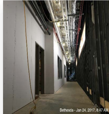
Dry wall installation in major corridors
